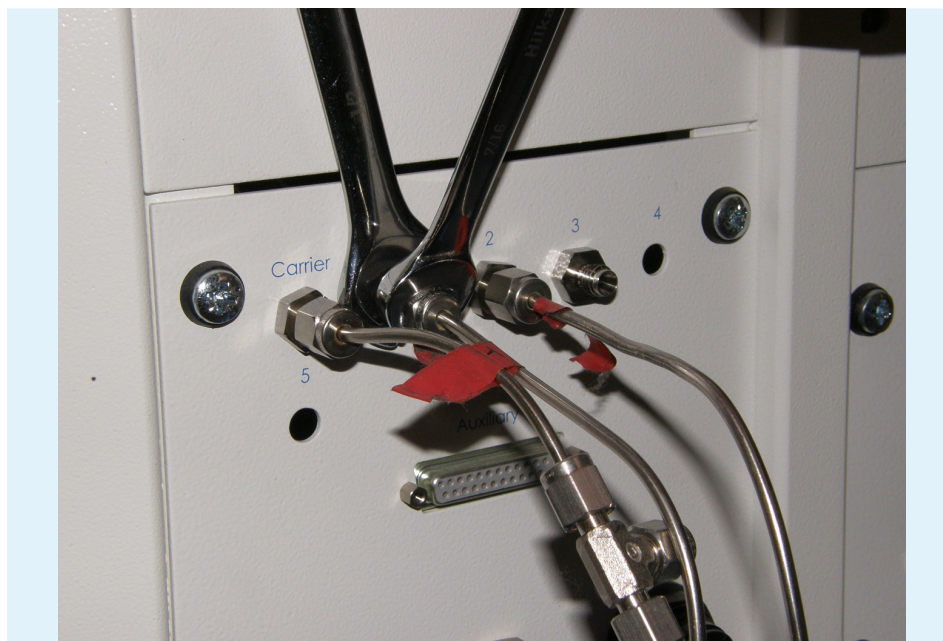
Figure 3.6-4: Purging the reference gas line.
